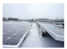
When installing solar power, there are a wide range of issues to investigate, including its impact on the outward appearance of the roof and its effect on the waterproofing layer. What we developed at that time was the drying foundation stand "PV-FIX" series. Through a reliable interaction with the waterproofing layer, we can support solar panels in a smart way. There is a rich lineup provided in combination with various waterproofing methods.
