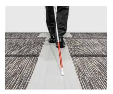
Tiles to guide the visually-impaired. These are increasing on sidewalks and stations, but once you set foot in a building there is only a legal requirement to install these as far as reception. The UD floor system is an item exclusive for indoor that minimizes the height of protrusions, and enables you to be guided safely within the building.
