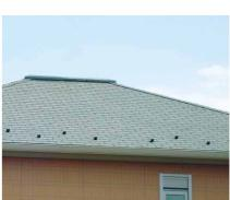
A wide variety of shapes, such as curved surfaces, multiple surfaces, and steep gradients, are required for sloped roofs that determine the form of the building. The asphalt shingle "Mitsuboshi Roarny II, Roarny II Square", which fully utilizes its light and flexible performance, supports all kinds of situations and enriches the expression of the roof.
