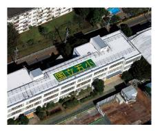
Disaster assistance helicopter providing supplies and aid from the skies during an emergency. The helicopter sign drawn on the roof is a landmark. Clear visibility is required in preparation for disasters that could occur at any time. "Flector film" has reliable retroreflective performance even at night, and provides visibility you can rely on for 24 hours.
