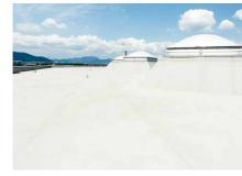
We have a product called "VIEW TOP" which is a method of creating a waterproof layer in which the roofing sheets use vinyl chloride resin as raw materials, are fixed in the foundations with adhesive and anchors/discs, and the sheets are mutually pasted together. And we also have "PLAST SHEET" made of vulcanized rubber sheet which has excellent weather resistance. Its features simplicity and shortness of construction period.
