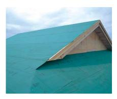
A roofing material that protects the roof of a detached house from rain leaks.
