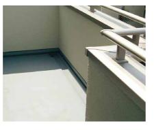
The waterproofing method for wooden structures is perfect for balconies in wooden houses. We have prepared a variety of methods, such as those using vinyl chloride sheet waterproofing "Roku-sheet", environmental-type urethane coating waterproofing "Patio-all", and FRP waterproofing with modified asphalt sheet "HOUTAN".
