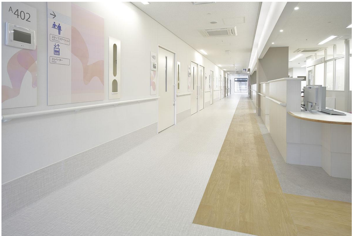
Flooring material raised up example
